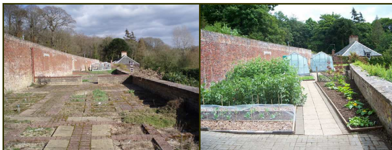
The walled garden terrace before work began and in mid-summer 2007
